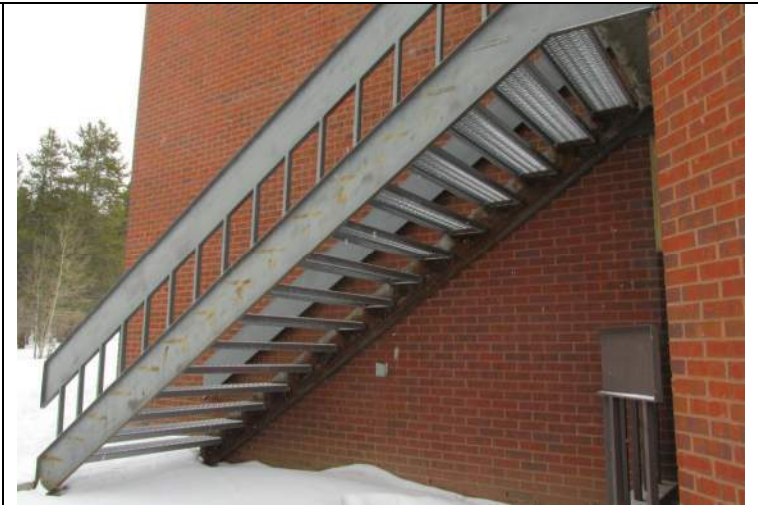
↑East wing (west side)
