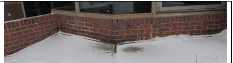
↑ Sill walls near aquatic center entry
