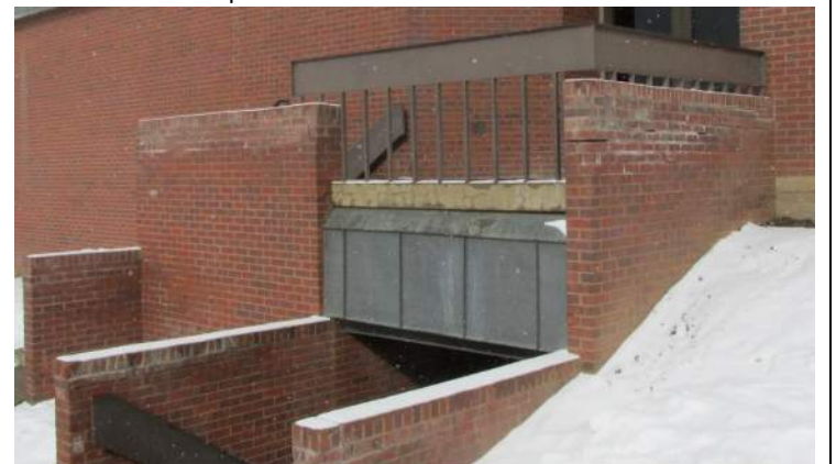
↑ Cantilevered walls at library entrance
