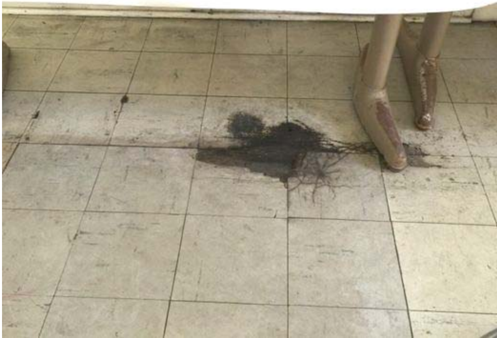
Asbestos tile mitigated by covering with real oak hardwood flooring, installed by FOTL.
