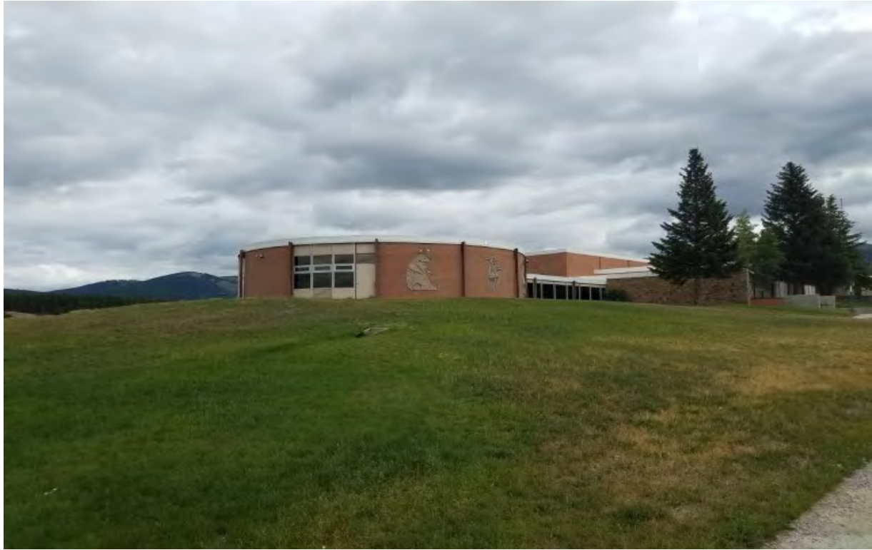
Photo 3. View of the west exterior of the school.
