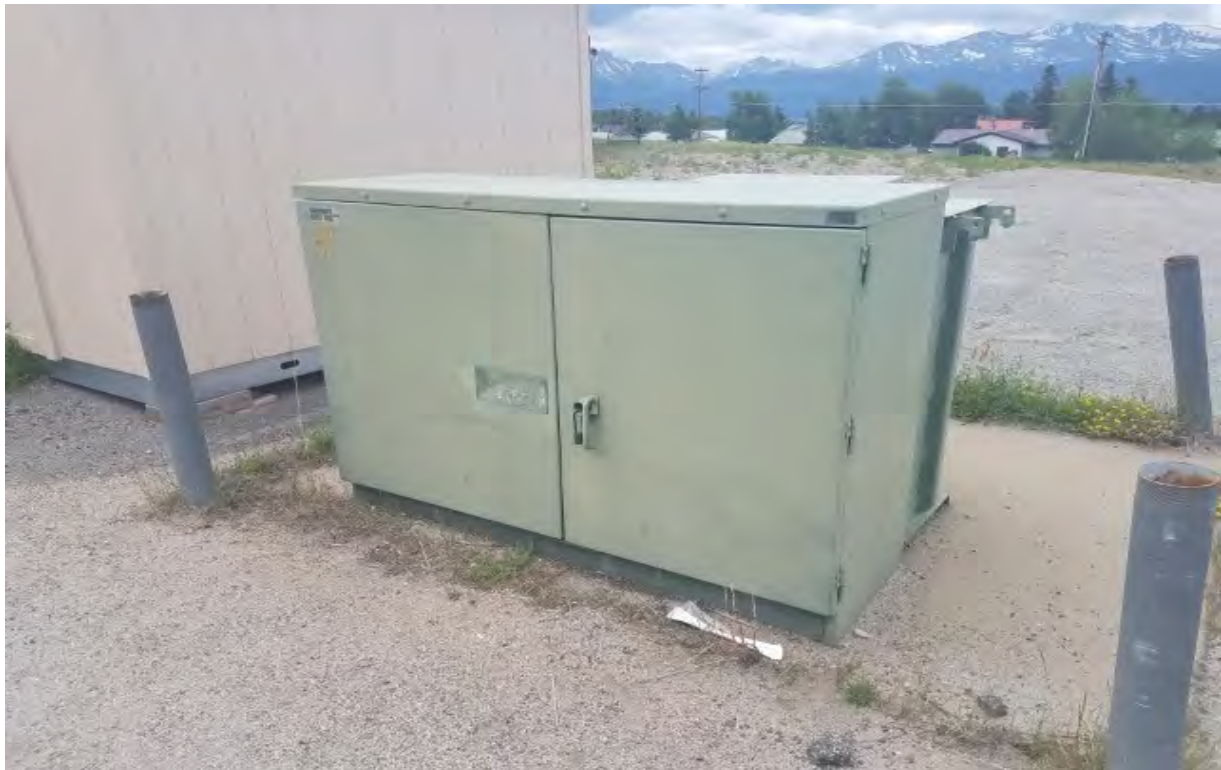
Photo 4. View of the pad-mounted transformer located on the site.
