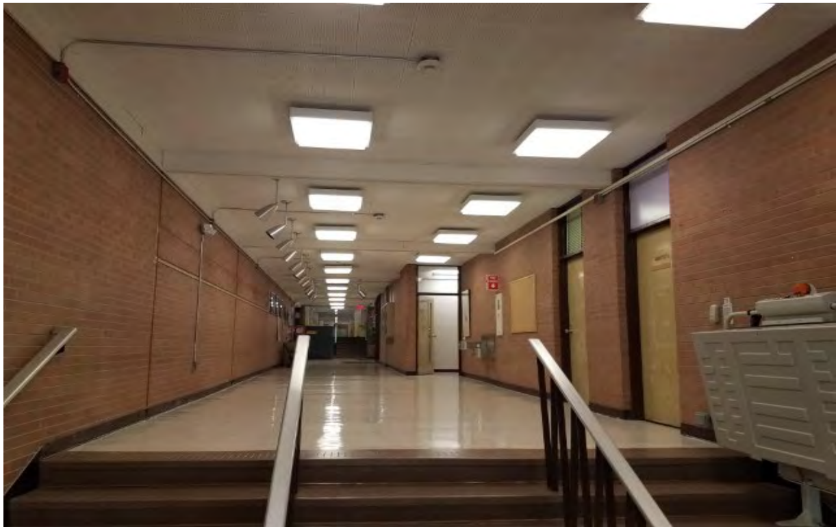
Photo 8. View inside one of the school hallways.
