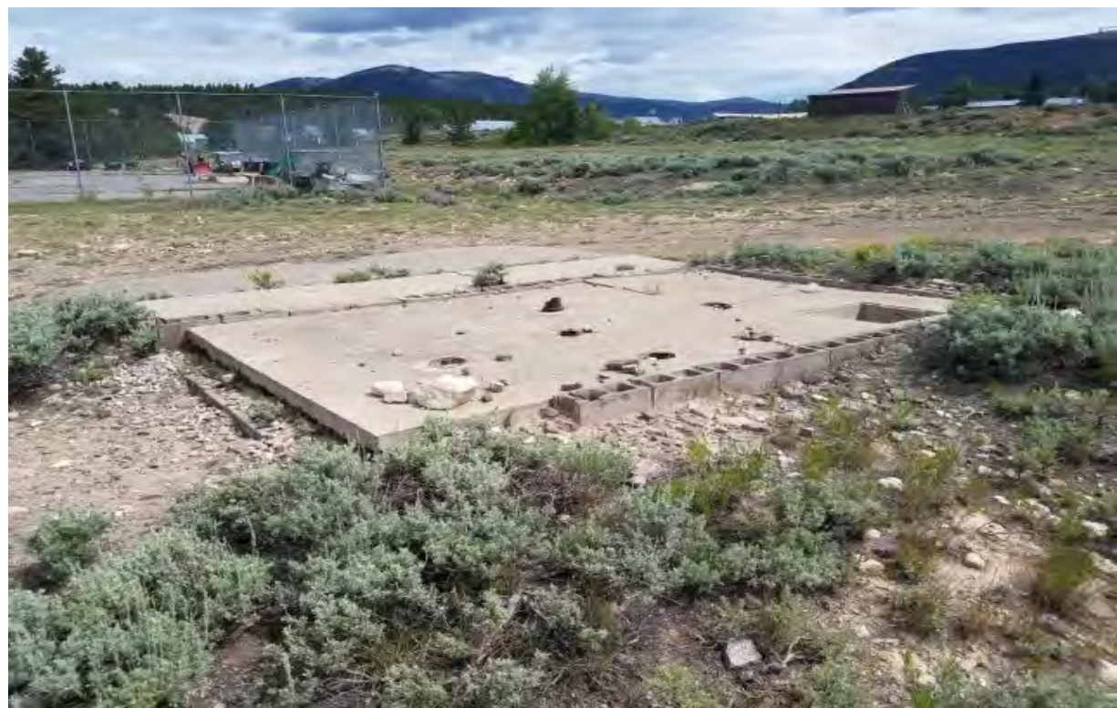
Photo 14. View of concrete slab near the north property boundary.
