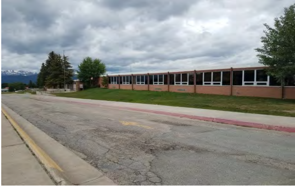
Photo 1. View of the south exterior of the school.
