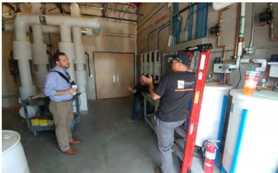
West Park Elementary School Replacement Project
