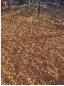
G2052 - Erosion Control Measures Site
