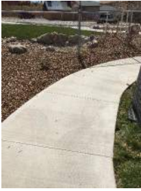
G2031 - Paving and Surfacing Site
