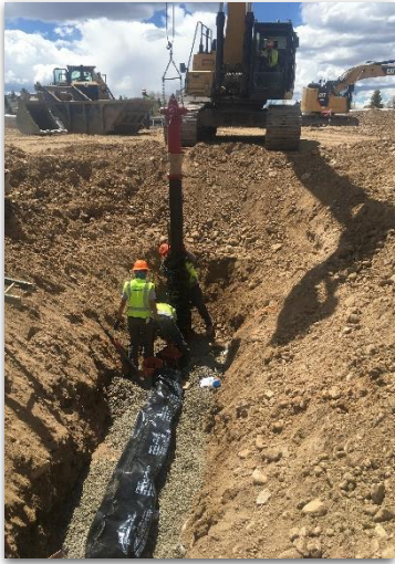
Fire Hydrant Installation
