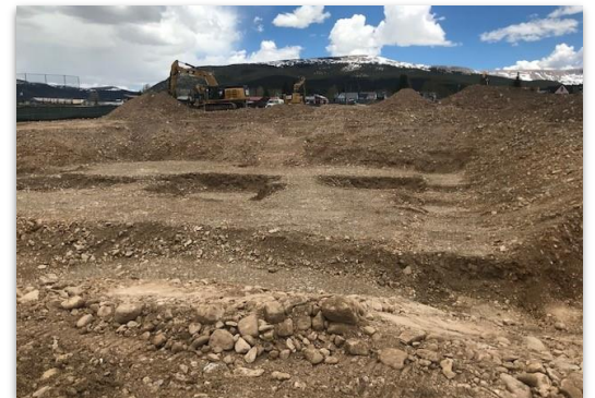
Basement and Footing Excavation
