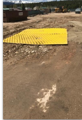
Tracking Pad Installation
