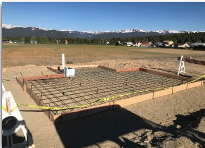
Formwork for the New Water Fill Station
