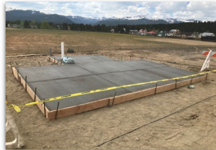
Poured Slab for Water Fill Station
