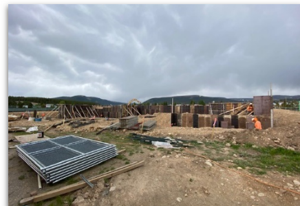
Wall Formwork
