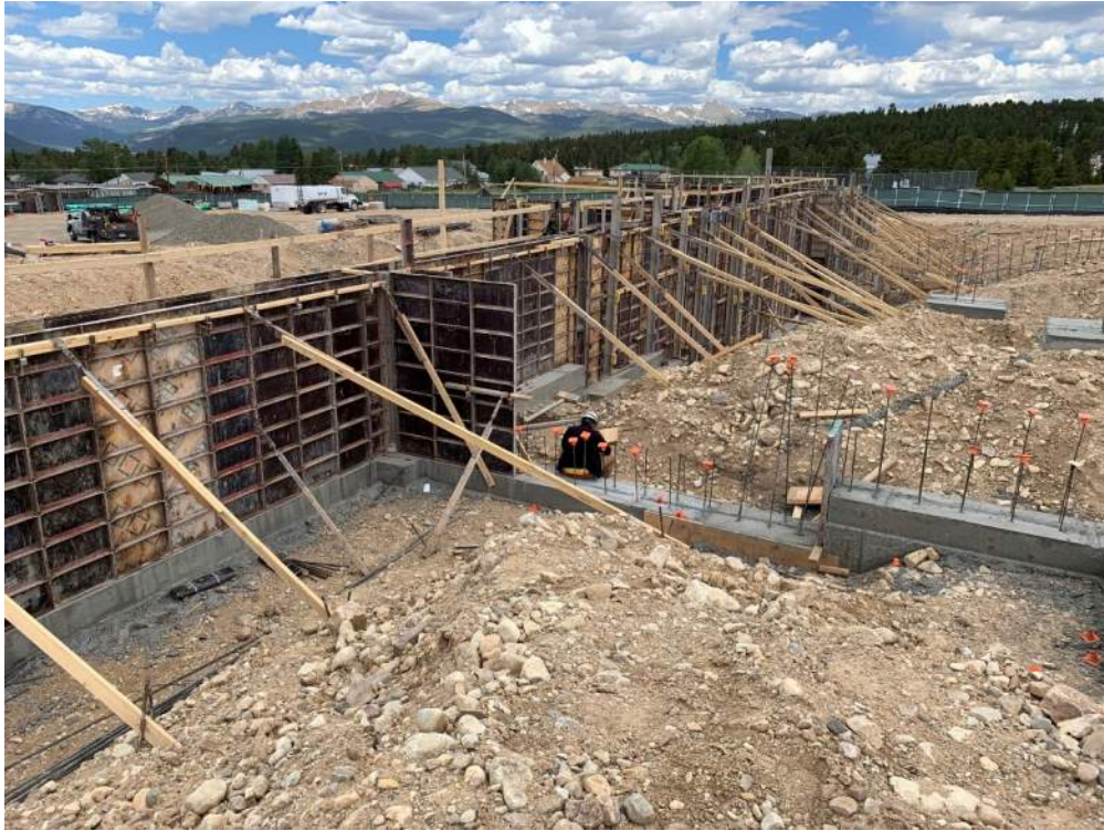
7/7/2020 – Foundation Formwork
