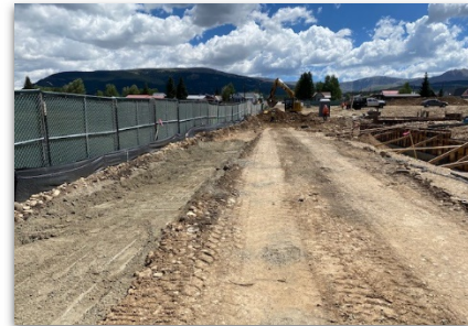
Curb and Gutter Prep
