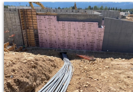
Underground Utility Installation
