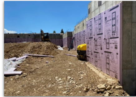
Area A Dampproofing/Waterproofing
