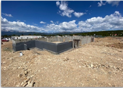
Area A Dampproofing/Waterproofing
