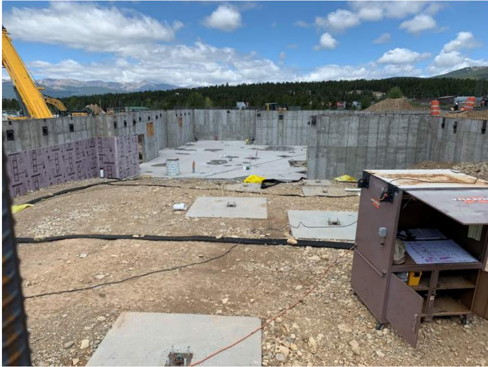
9/1/2020 – Mechanical Basement Concrete Slab
