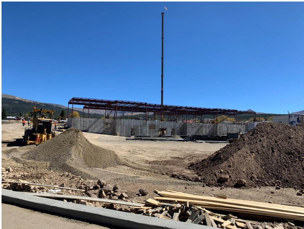
9/30/20 – View from the curve of the parent drop off access road
