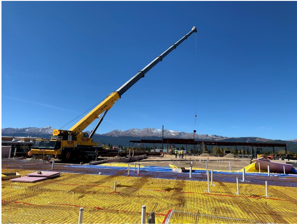
9/30/2020 – View from east wing
