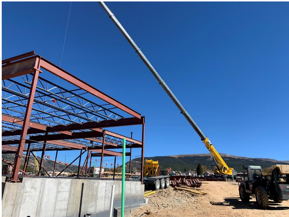
9/30/20 – Steel erection of west wing
