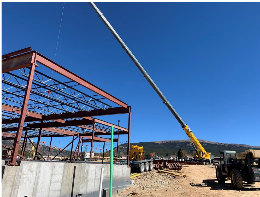
9/30/20 – Steel erection of west wing
