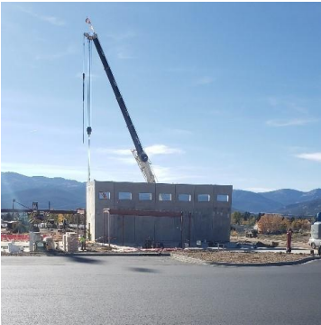
PRECAST GYM PANELS & UPPER LOT PAVING
