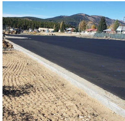
UPPER LOT PAVING
