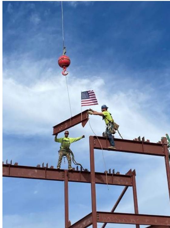
11/3/2020 – Topping Out Beam
