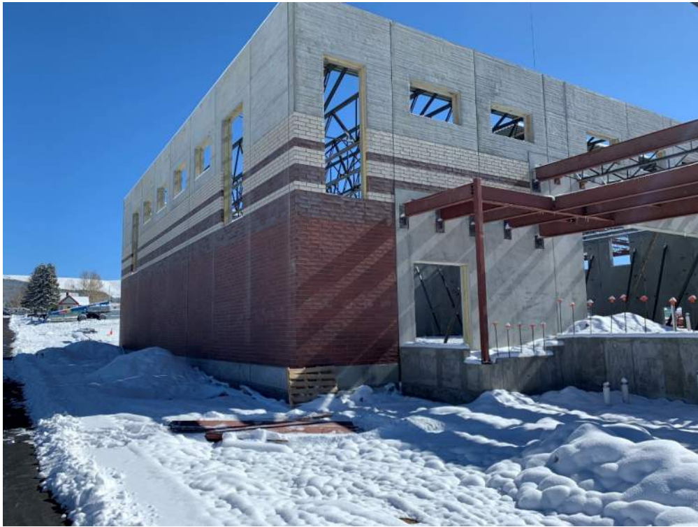
10/27/2020 – Exterior of Precast Gym
