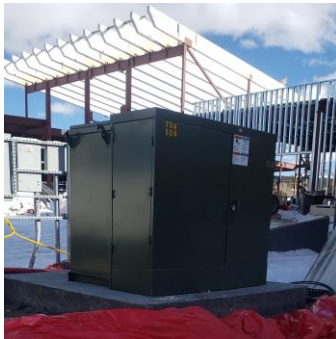
TRANSFORMER INSTALL
