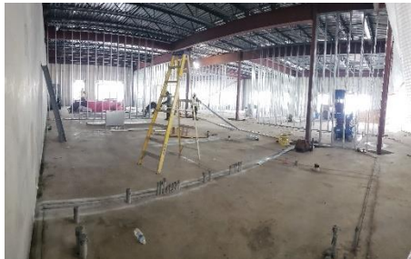
INTERIOR FRAMING AREA B
