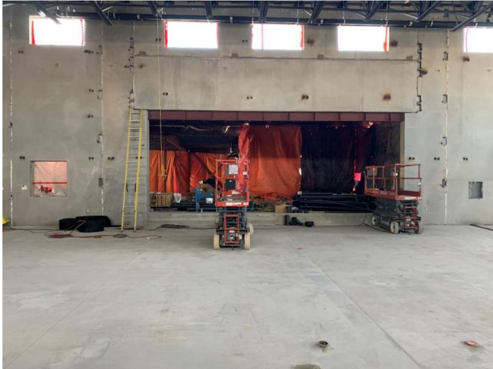
12/22/2020 – Stage Opening to Gym
