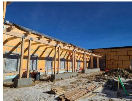
CANOPY FRAMING COMPLETE
