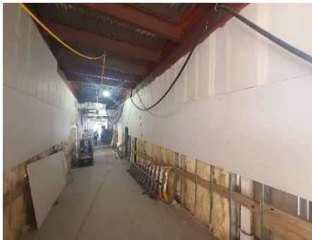
AREA A CORRIDOR DRYWALL & DUCT
