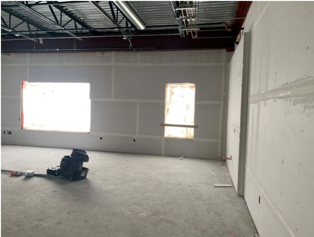
1/26/2021 – Drywall in Classroom
