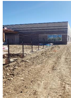
OUTDOOR LEARNING FENCE POST INSTALL
