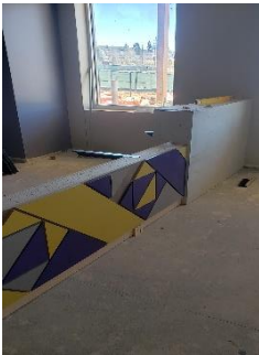
ADMIN CASEWORK INSTALL
