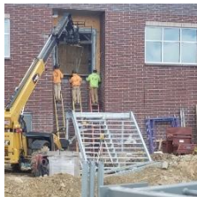
WEST STAIR INSTALL
