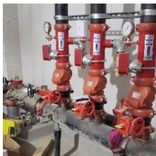
FIRE RISER ENTRY
