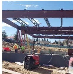
ADDITION IRON ERECTION
