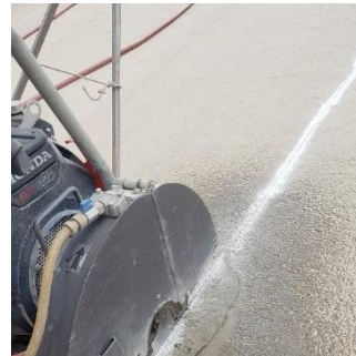
CURB AND GUTTER ASPHALT CUT @ DRIVE LANE
