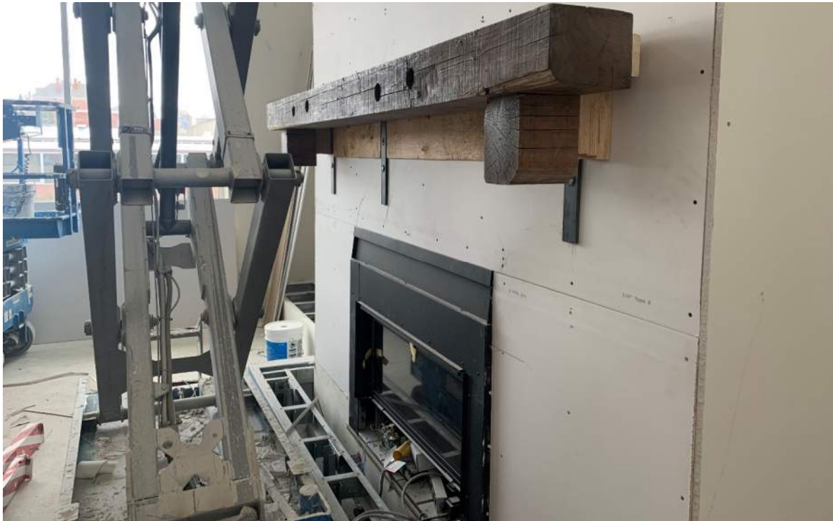
6/1/2021 – Media Center Fireplace Mantel
