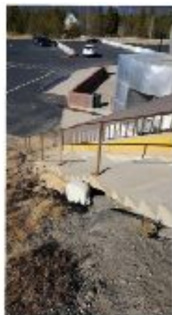
COMPROMISED EXTERIOR CONCRETE STAIR
