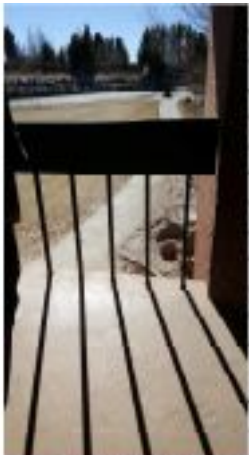
EXTERIOR STAIRS AND RAILINGS - NON CODE COMPLIANT
