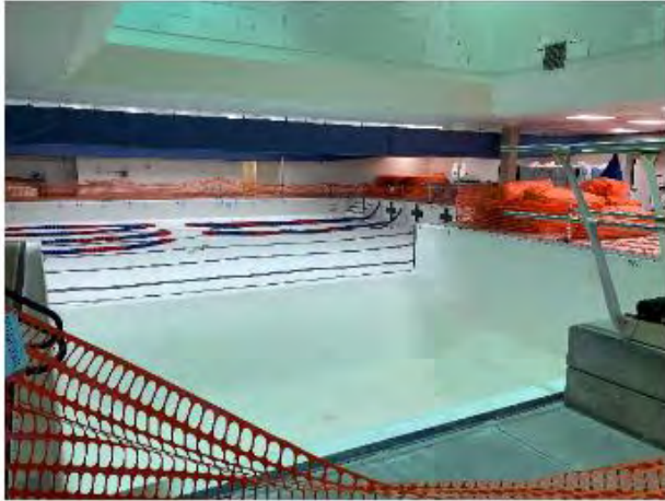
Image 1: Overall View of the Pool
