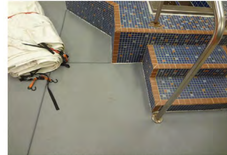
Photo 3: Surface coating on concrete slab
