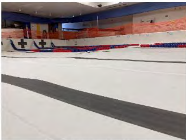
Image 5: Warped Pool Floor
