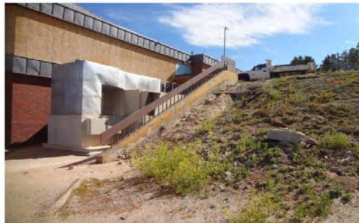
Photo 1: Exterior stairway has been removed
